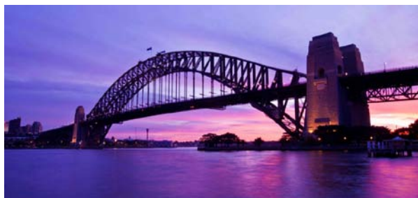
Fig. 4. Sydney Harbour Bridge [15]
